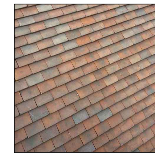
Clay Plain roof tiles to match existing style of tile seen on Farm House.
