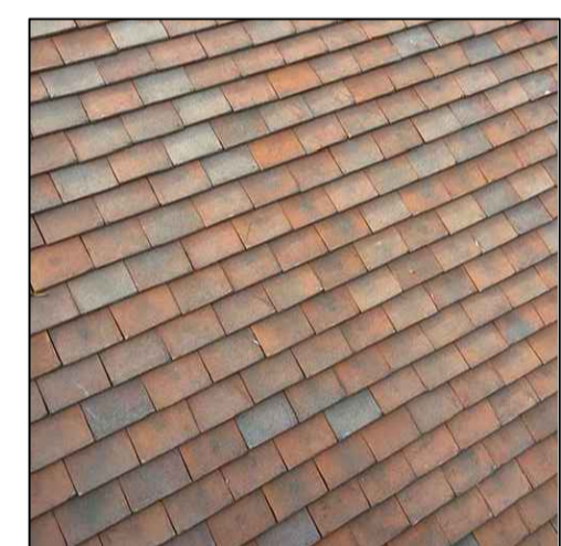
Clay Plain roof tiles to match existing style of tile seen on Farm House.
